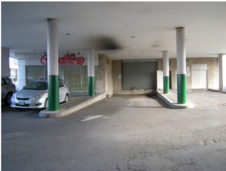
Figure 3.19: Shared loading dock facilities at a strip mall
