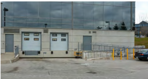
Figure 3.4: Loading dock ramp
