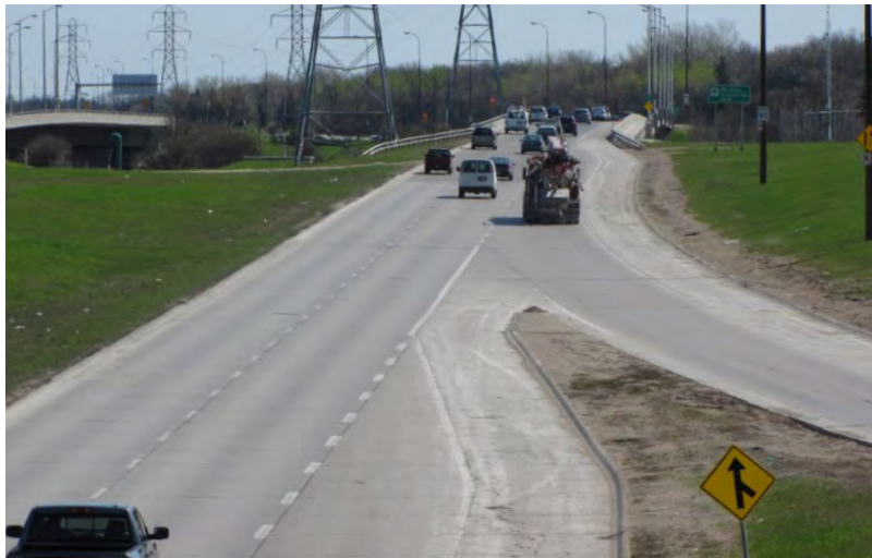
Figure 4.1: Acceleration lane on a major through corridor
