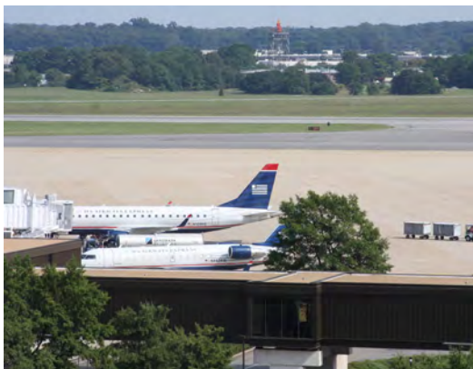
Figure 6.3: Norfolk International Airport, Virginia
