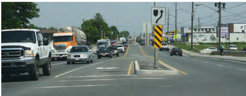
Figure 4.17: Narrowed lanes and lanes that have been restriped to add capacity
