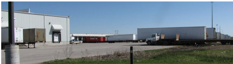
Figure 4.26 : Installation de transbordement
