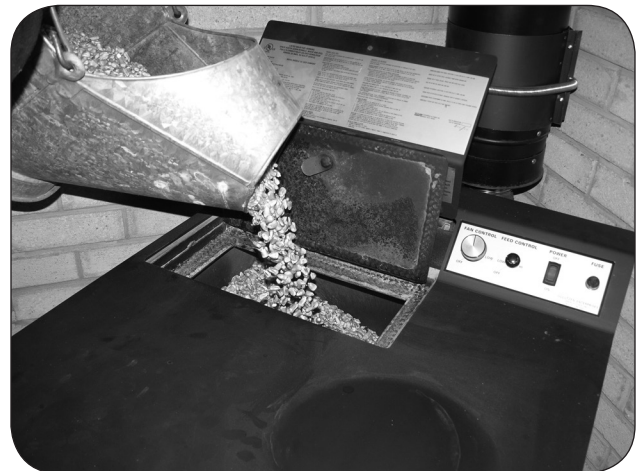
Figure 2. An old coal scuttle can be used to refill the fuel hopper located at the back of this stove.
