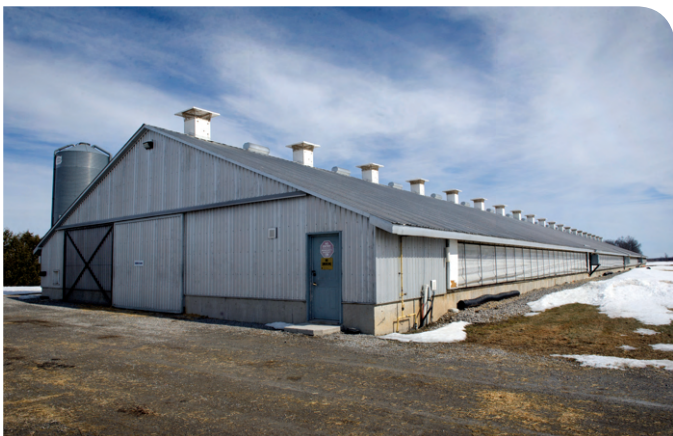
Figure 26. Exterior of a turkey barn.
