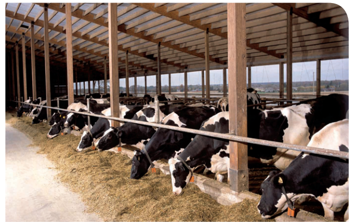
Figure 12. Interior of a free stall dairy barn.*
