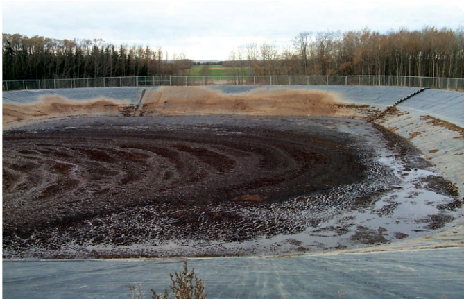
Figure 44. An earthen manure storage ; note the sloped sides and no cover (H1).
