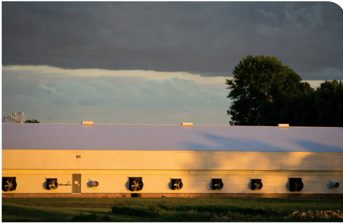
Figure 18. Exterior of a chicken layer barn.*
