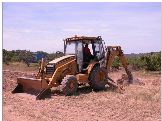
Figure 8. Digging a burial pit using a backhoe.
