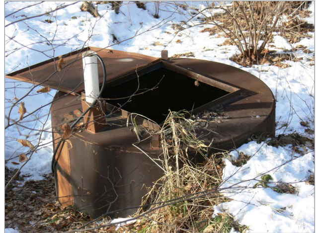
Figure 7. In-ground disposal vessel, with vent pipe and open hatch.
