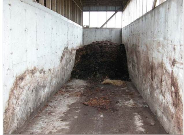
Figure 4. These concrete walls are 2.4 m high (8 ft) but the compost is never piled deeper than 1.8 m (6 ft). If building again, the operator would have made the bin 0.6 m (2 ft) wider than his loader, as it is a tight fit in a long, narrow bin like this.
