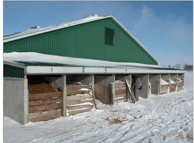
Figure 2. Bin system showing two primary and secondary bins, plus bins for finished compost and storage of substrate.
