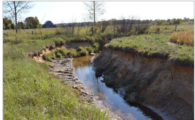
Figure 6. Bank erosion involves the undercutting and scouring of natural stream and drainage channel banks.
