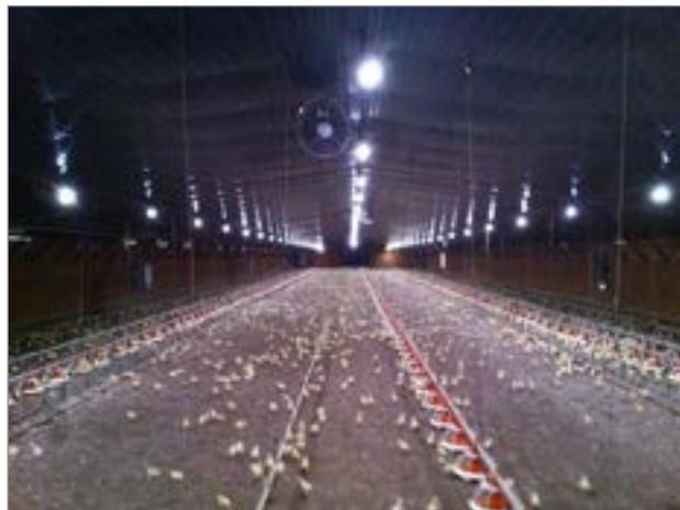
**Figure 5.** A poultry barn with 12W LED lighting spaced at 3.6 m (12 ft). Source: [www.poultryventilation.com](http://www.poultryventilation.com).
