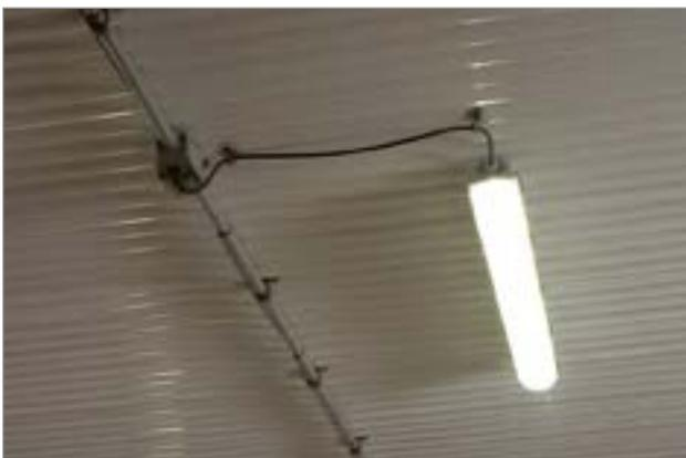
**Figure 10.** A tube LED enclosed fixture. The tube LED replaces a former T8 fluorescent tube using the same fixture.
