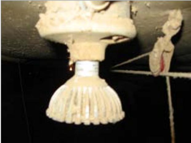
**Figure 8.** A different model of a finned LED bulb covered in a layer of dust. *Source:* National Poultry Technology Center, Auburn University, [www.poultryhouse.com](http://www.poultryhouse.com).
