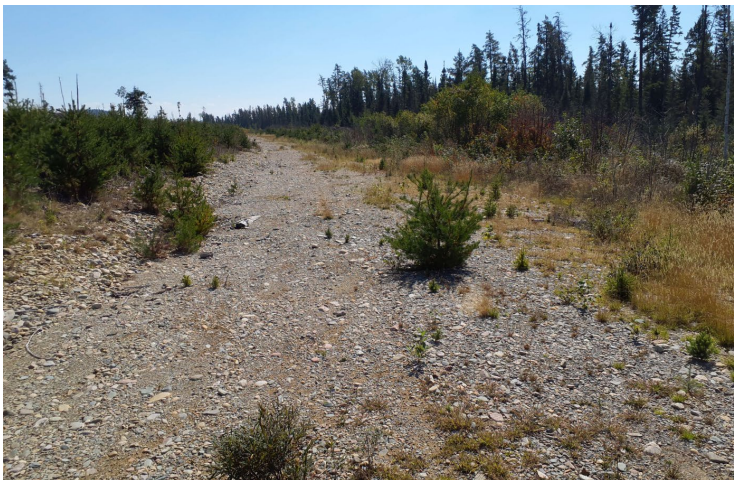
Kimberly 142 – Operational road in a harvest block. The road is regenerated and no longer drivable but 2023 A.W.S. list it as an existing road.
