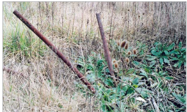
Figure 4. Surfaced well pipes.
