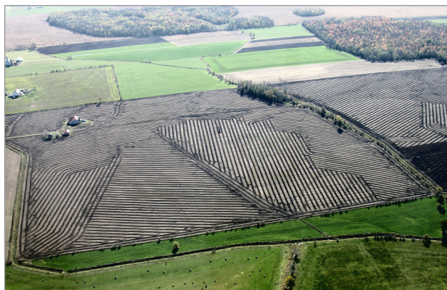
Figure 1. An aerial photograph of a field where tile drainage was recently installed.
