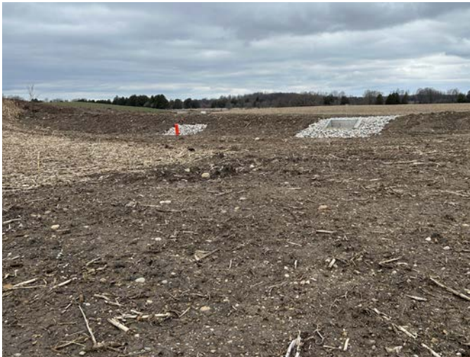
Figure 7–11. A constructed berm with multiple outlets designed to temporarily store water on the landscape. Source: Streamline Engineering Inc.
