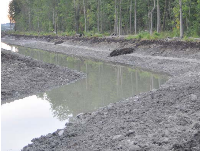
Figure 7-4. A dewatered channel with a littoral shelf on the right side of the channel.
