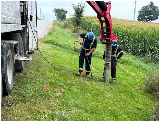
Figure 2–9. Example of increased costs required at a road crossing due to hydro excavation of utilities. Source Streamline Engineering Inc.
