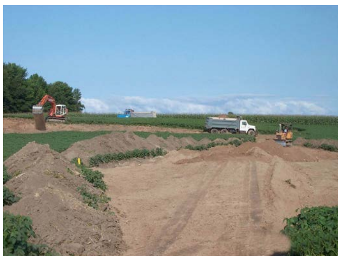
Figure 2–7. Damage to a soybean field resulting from drain construction.
