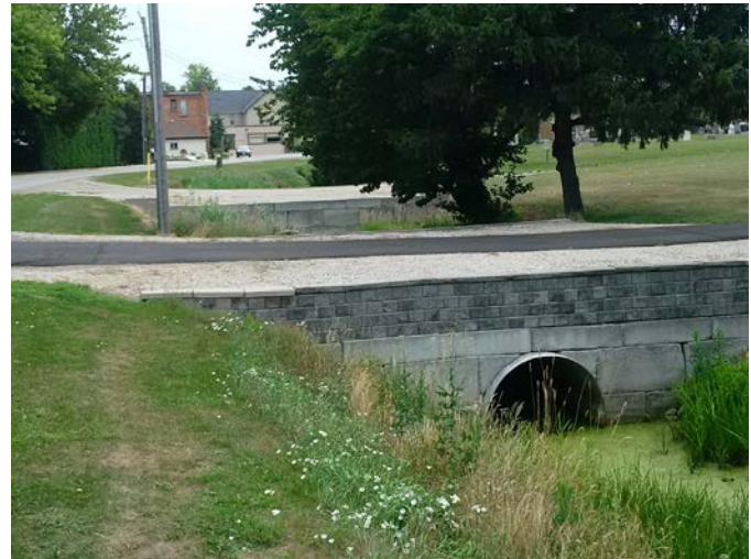
Figure 2–8. A crossing with decorative end walls. Source: Municipality of Chatham-Kent, Ontario
