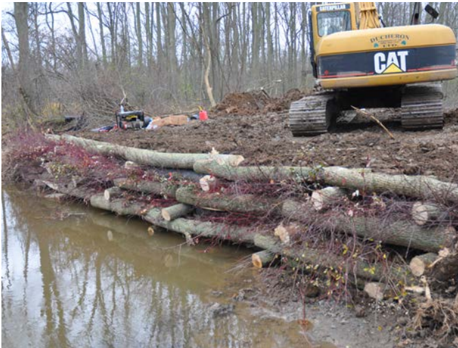
Figure 7-8. Construction of a live crib wall.
