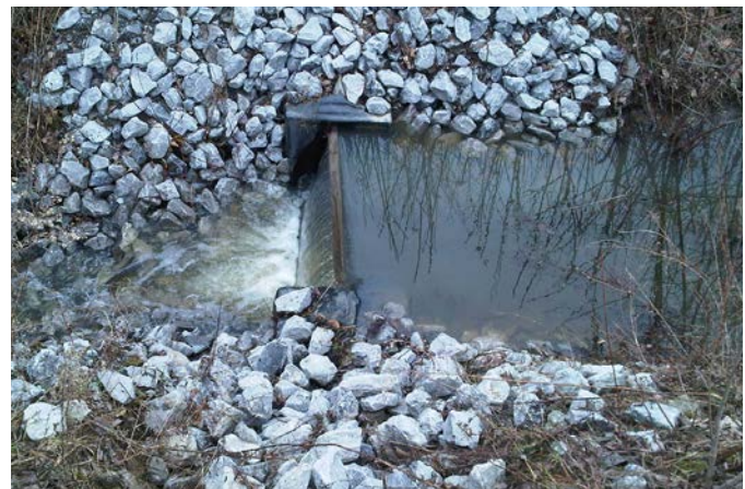
Figure 7-10. A water control structure.
